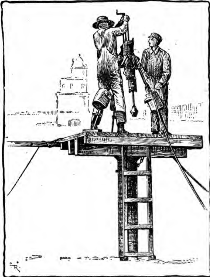
Fig. 175. View of Portable Drill Platform with Drill Mounted and Ready for Operation.
